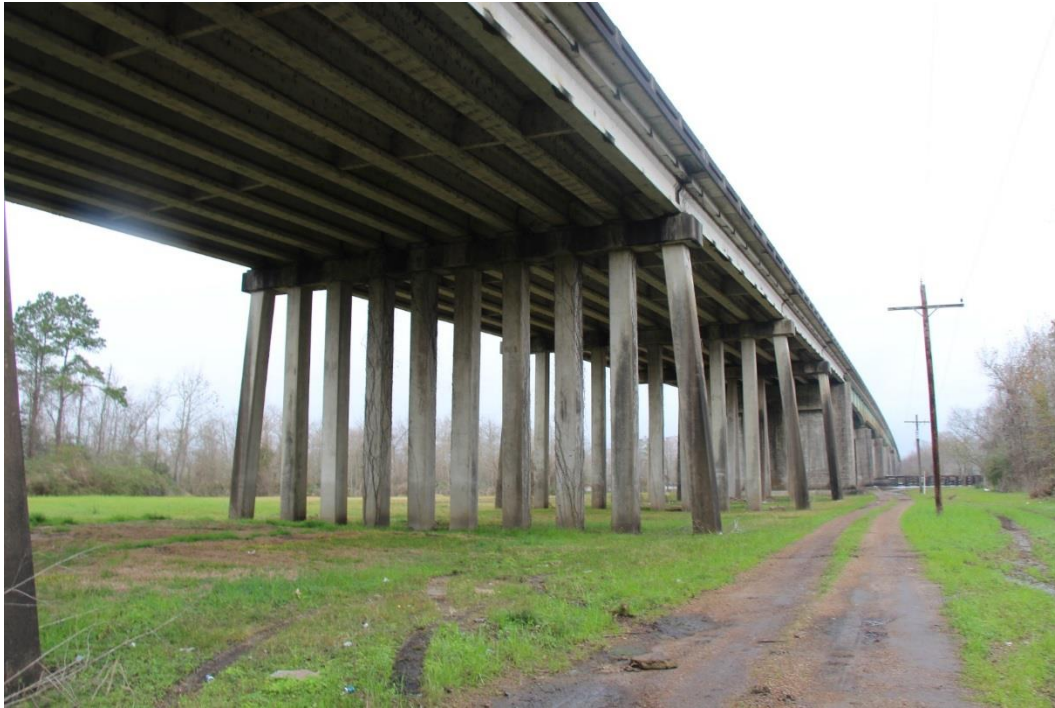
Condition Photo 7: Elevation view of concrete bents of the approach spans.
