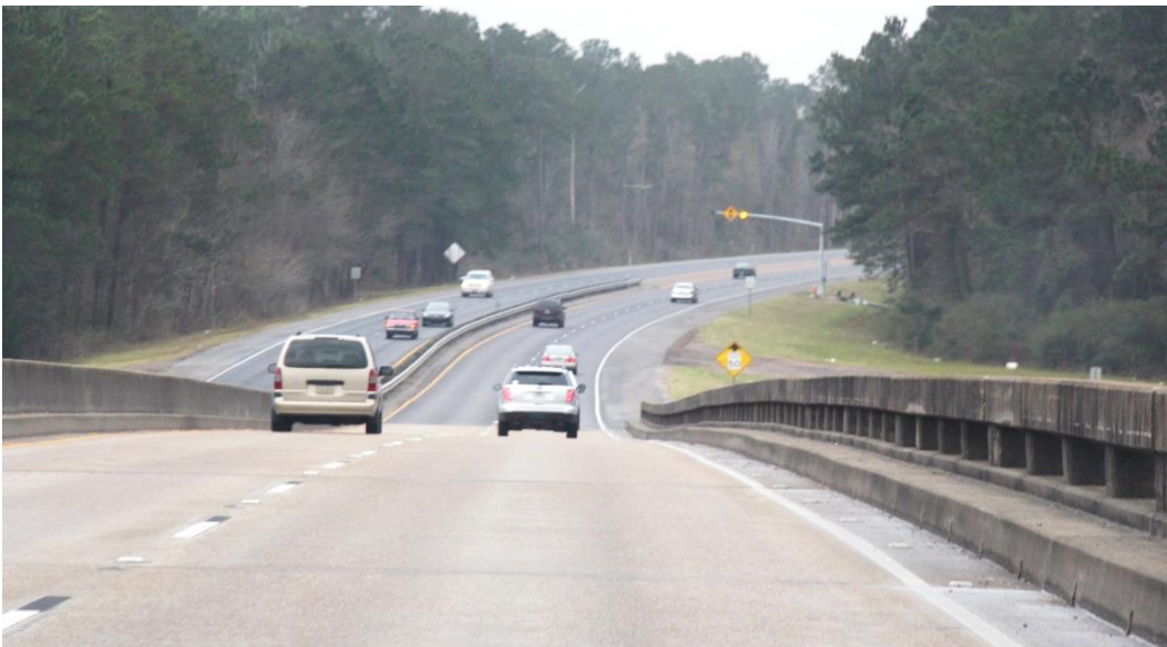
Condition Photo 2: Southbound travel lanes, looking south at south end of bridge.
