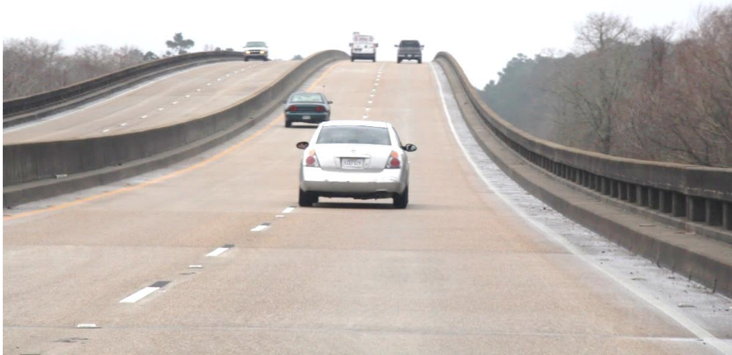
Condition Photo 3: Approach spans concrete deck slabs, looking north.
