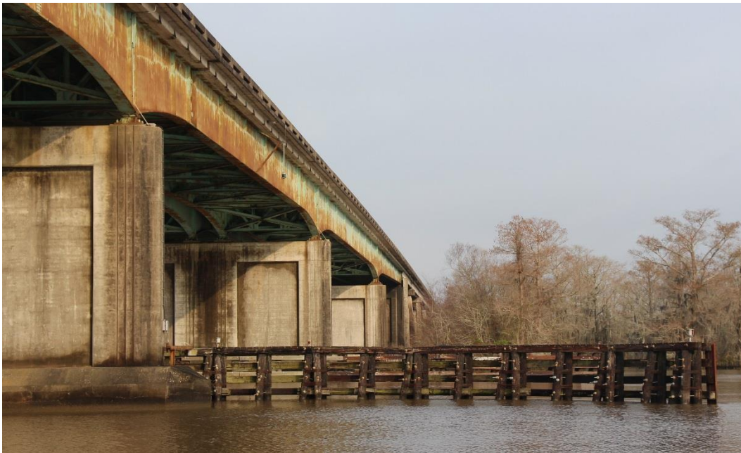
Historic Fabric Photo 2: Concrete piers for main steel plate girder spans.
