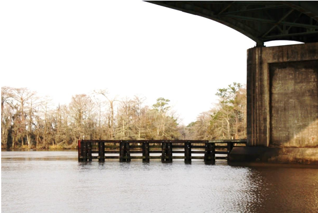
Condition Photo 17: West timber fender system.
