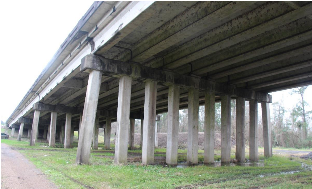
Historic Fabric Photo 1: Concrete bents for approach spans.
