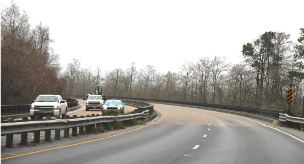
Condition Photo 1: Southbound approach, looking south at north end of bridge.
